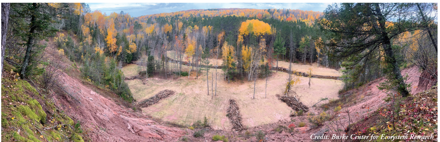
North Fish Creek sediment reduction project completed in the Town of Keystone, Wis.
